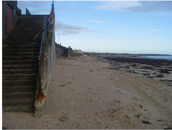
Plate 8 – Survey photograph 1aNTDC04A_20120928_N1.jpg
