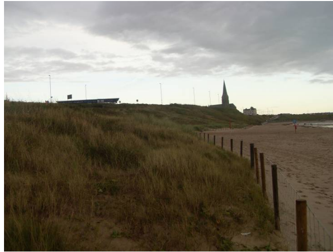
Plate 10 – Survey photograph 1aNTDC06A_20121002_N6.JPG
