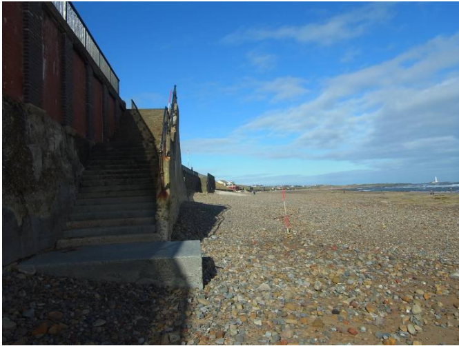
Plate 7 – Survey photograph 1aNTDC04a_20130312_N1.jpg
